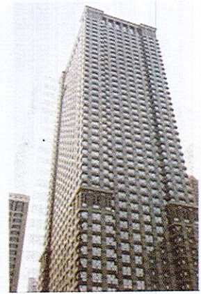
LEO BURNETT BUILDING, CHICAGO, MỸ
