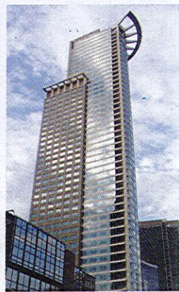
DG BANK, FRANKFURT AM MAIN, ĐỨC
