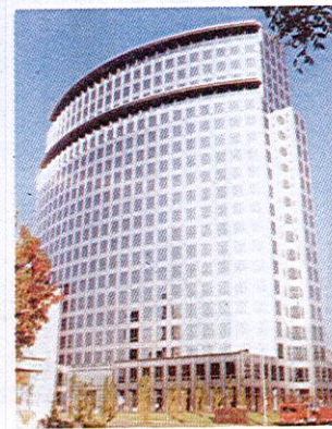
PLAZA TOWER, CALIFORNIA, MỸ
